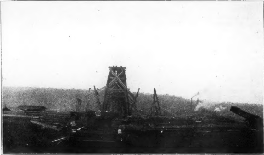
Tunnel Which Will Run Under Stock Pile
